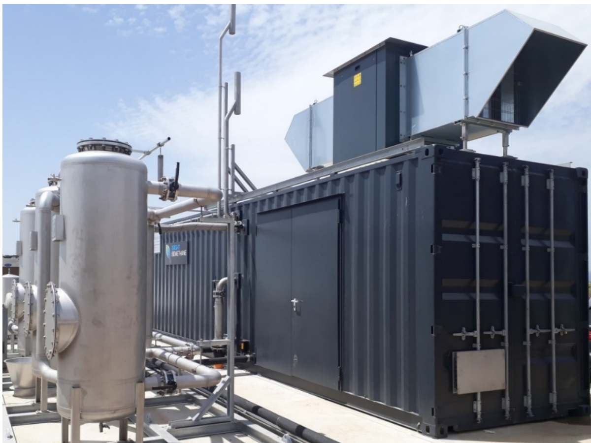
Illustration2. Membrane upgrading unit
